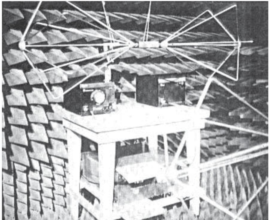
Figure 13. Electromagnetic interference immunity test setup.
