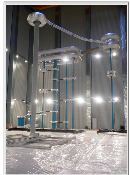
Type Test According IEC 60 at High Voltage Laboratory During withstand voltage test at +1200 kV DC
