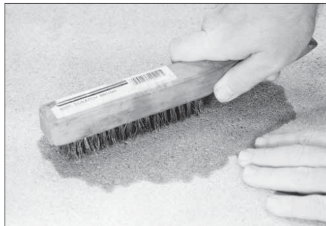
Figure 1 – Conditioning the surface for gage installation.
